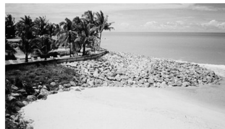
Rock rubble - Santubong, Malaysia (designed by WRL)
